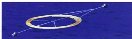
Figure 1. 120 m floating spiral for an 8 in. pipeline.
