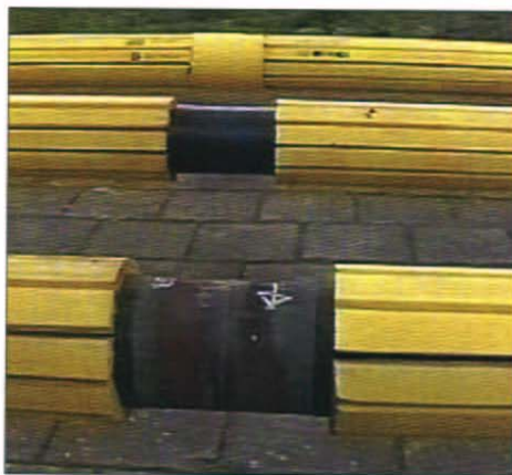
Figure 2. Strips of foam welded to the pipe make the pipe buoyant when launched.
